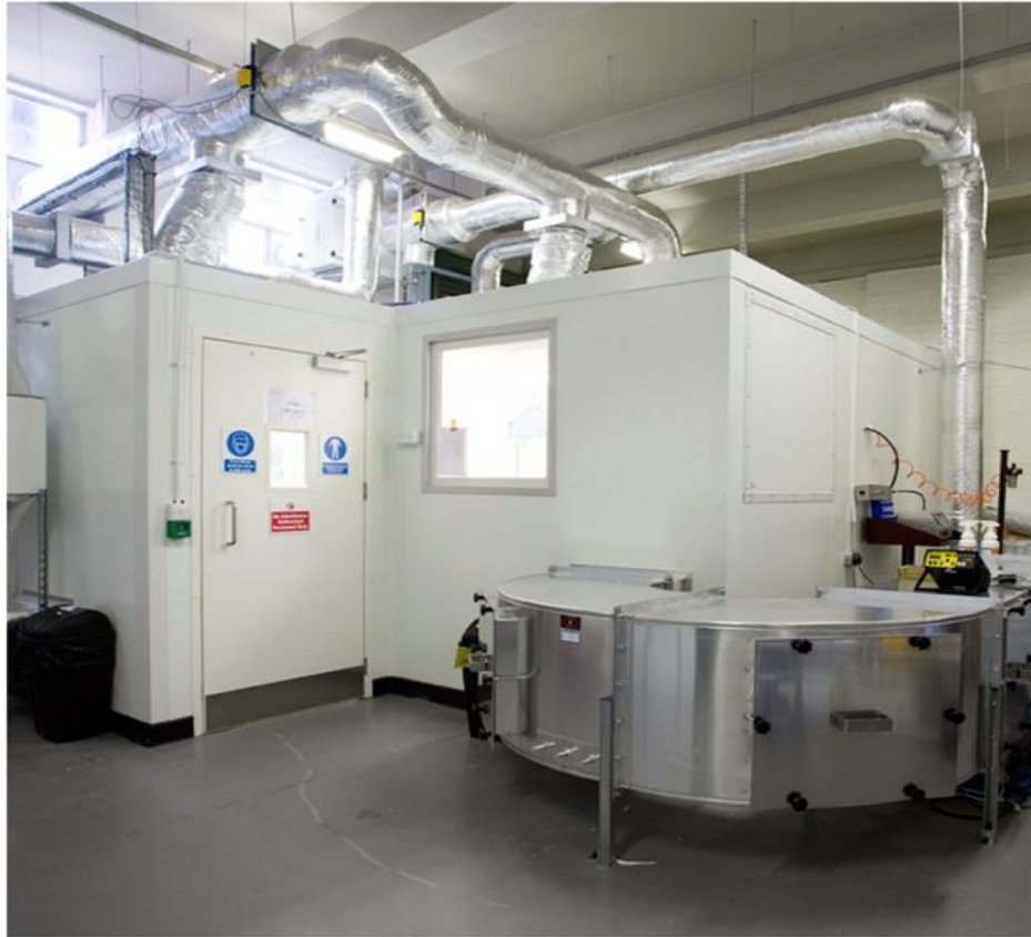
Figure 1: 28.5m 3 chamber and adjoining modified ASHRAE 52.2 test duct
